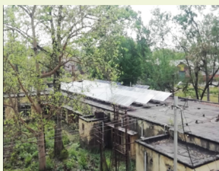
Pictures Showing Installed Roof Top Solar Plant (25 KWP) installed in Central WorkShop, Barkakana
