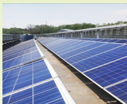
Pictures Showing Installed Roof Top Solar Plant (400KWP) in CCL Head Quarter
