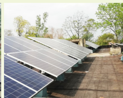
Pictures Showing Installed Roof Top Solar Plant (25 KWP) installed in Central WorkShop, Barkakana
