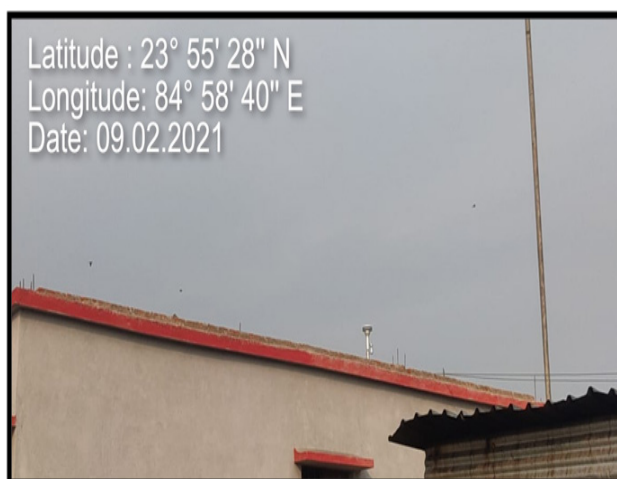
Continuous PM10 analyser installed at Railway Sidings of CCL
