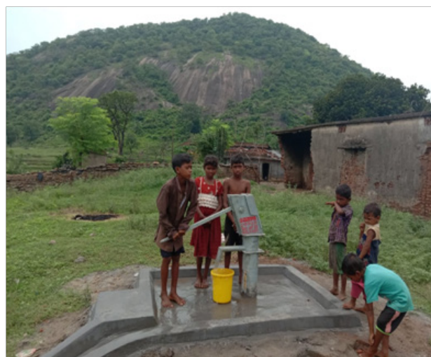
Handpump installed at Birhor Basti, CRS Barkakana
