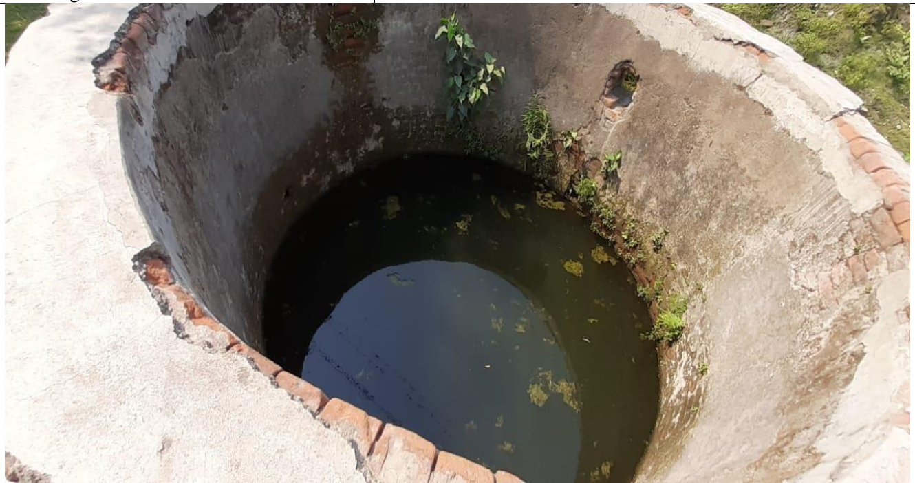
Piezometric Well near Dhori Khas (UG) Mine
