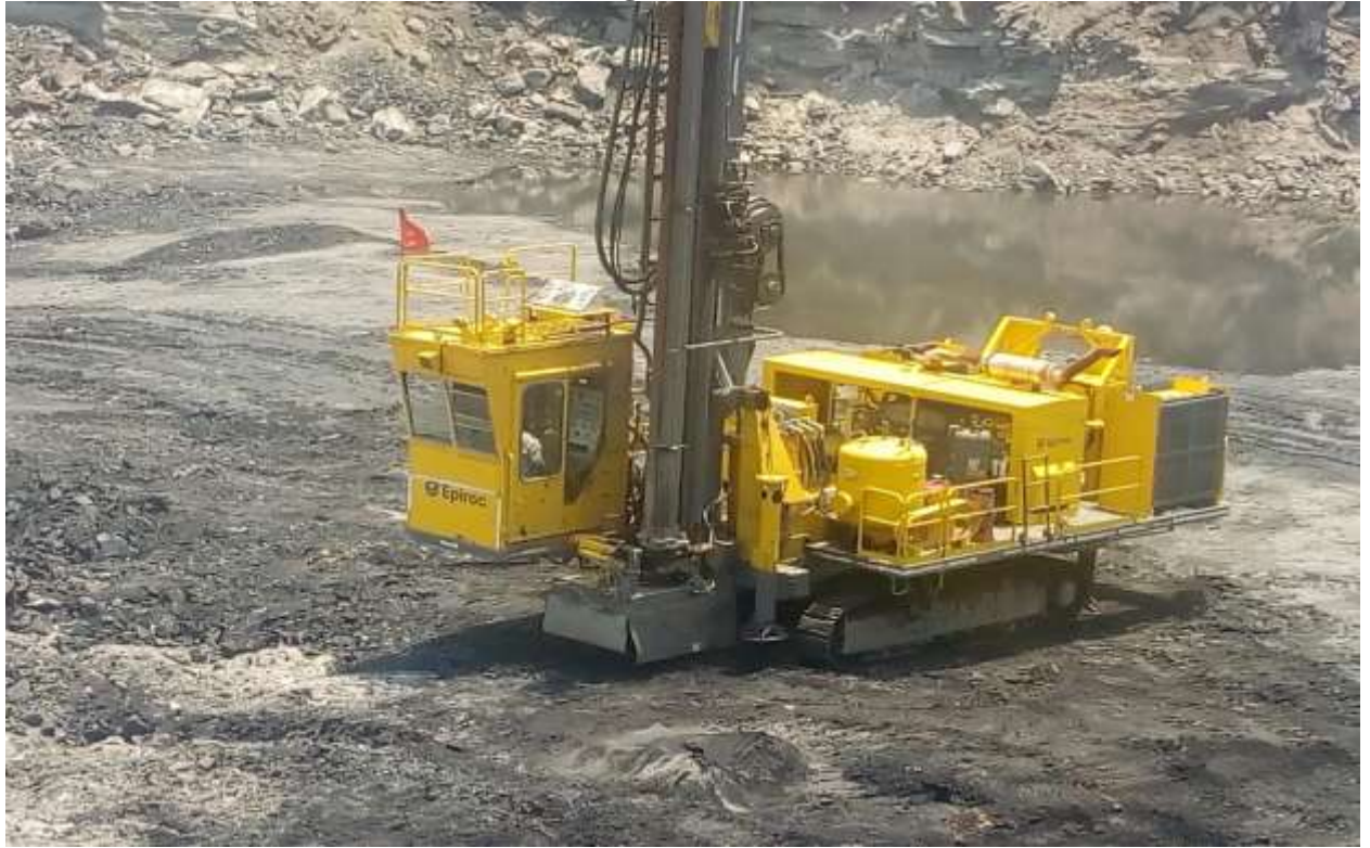
Wet drilling at Rohini OCP
