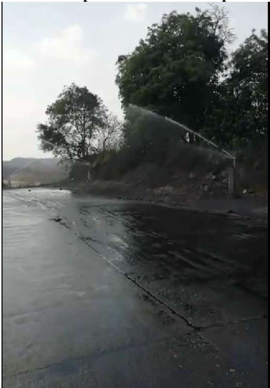
Fixed water sprinklers in Coal transportation road
