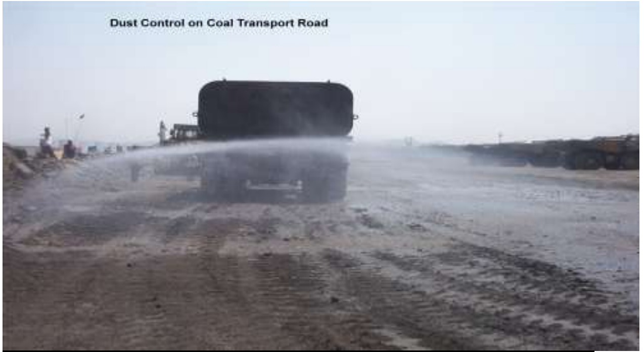
Water Sprinkler on haul road of Rohini OCP
