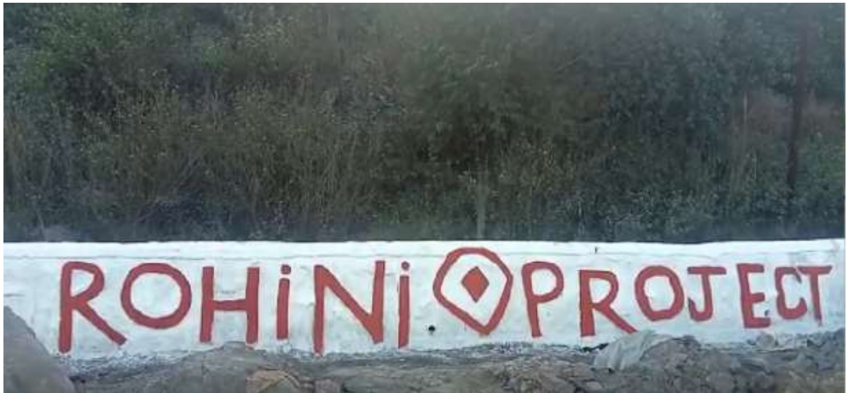
Toe wall/ retention Walls in Rohini OCP
