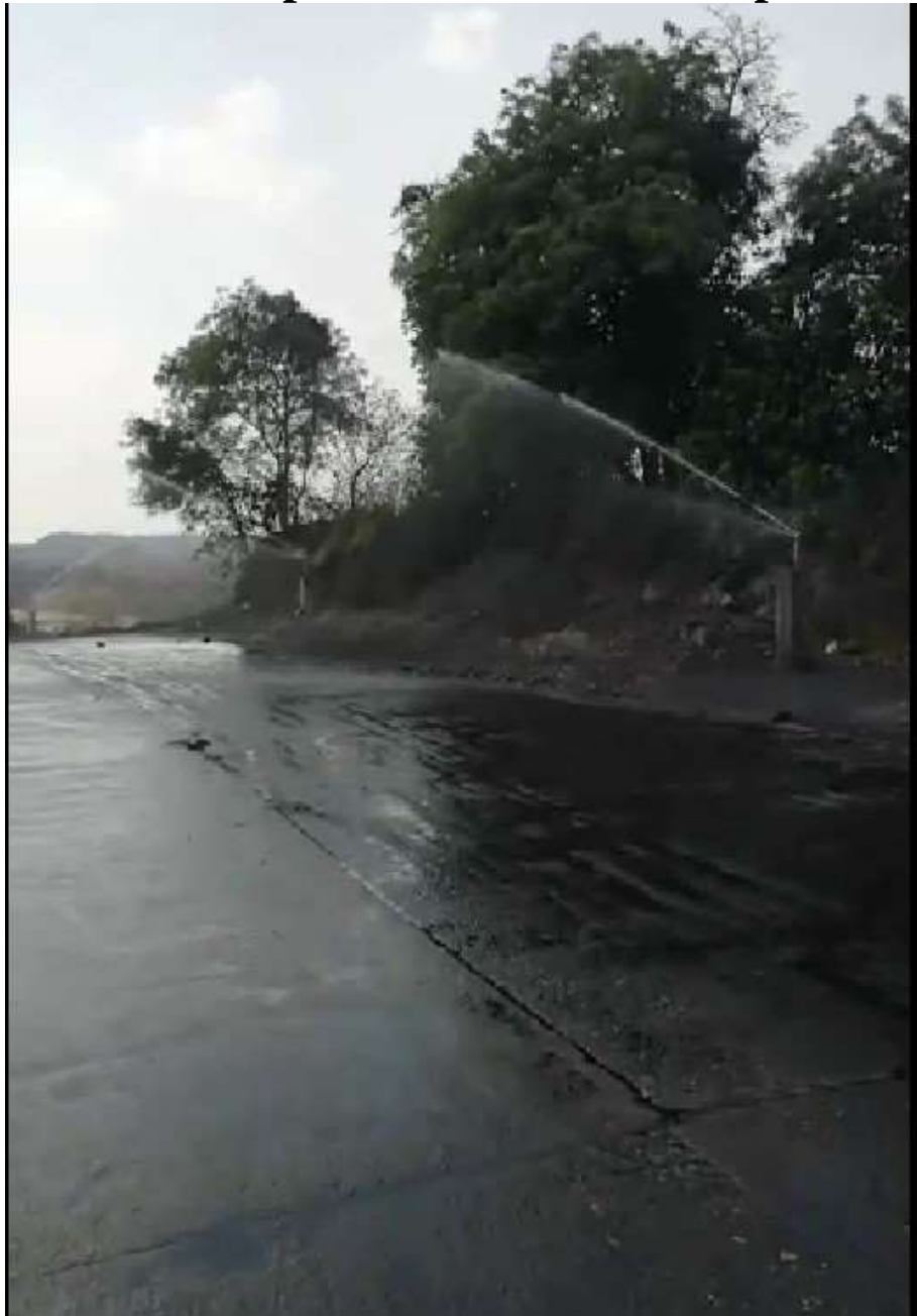
Fixed water sprinklers in Coal transportation road
