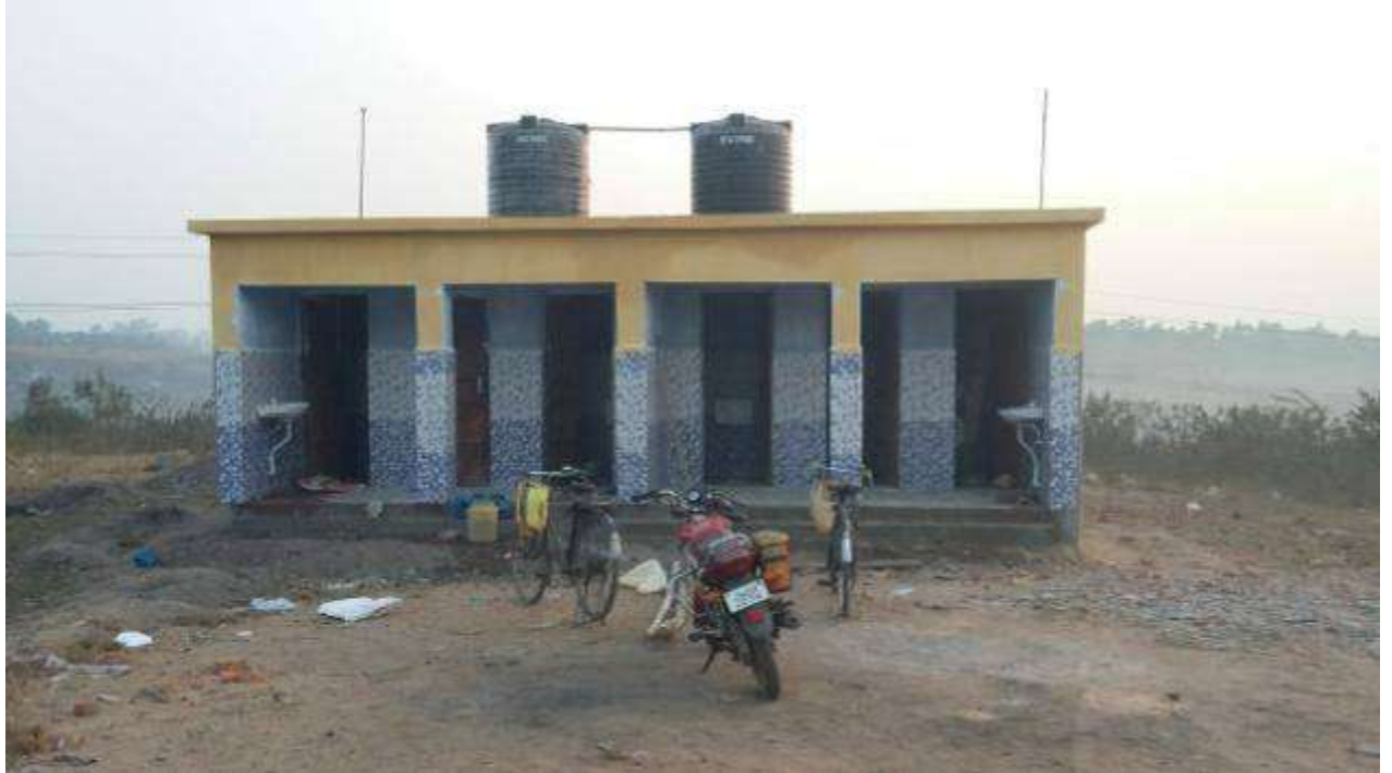
Construction of toilets
