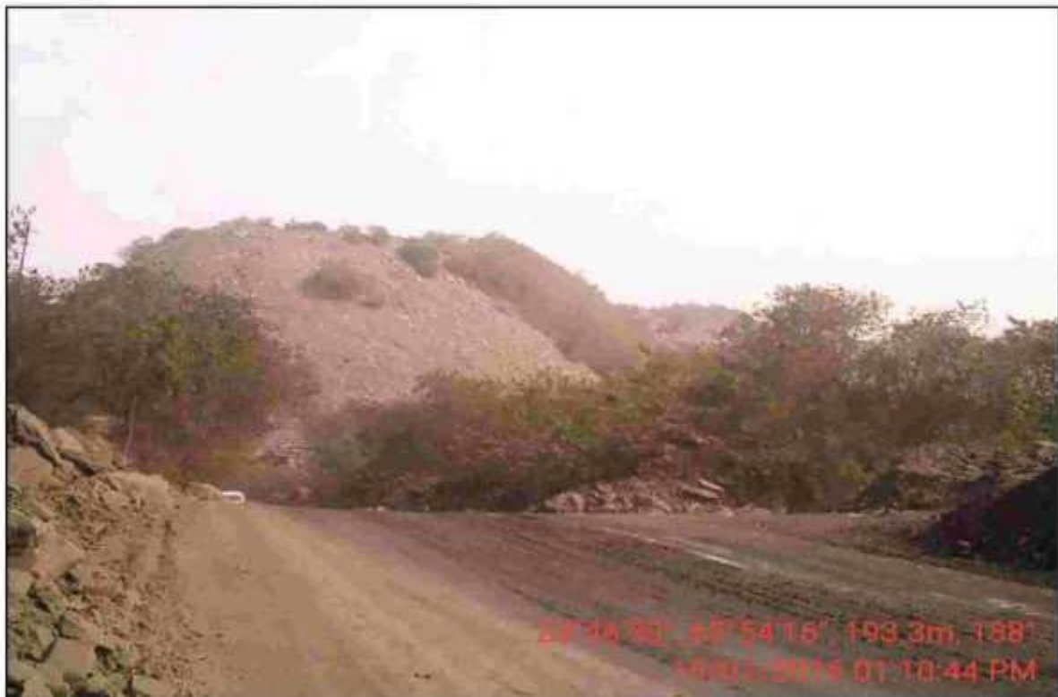
Photo 7: Plantation on Backfill (Jarangdih OCP)
