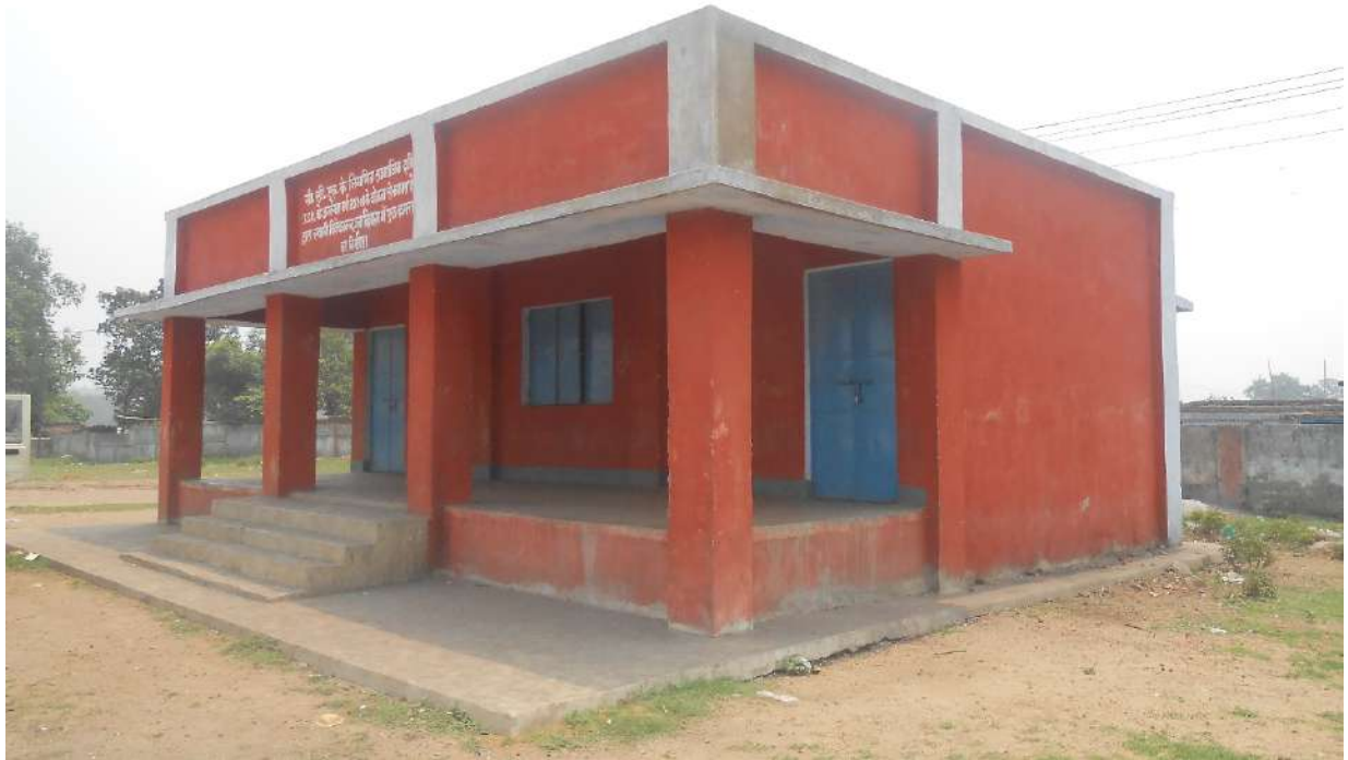
Figure 13: Construction of Classroom at Vivekanand High School, Jarangdih
