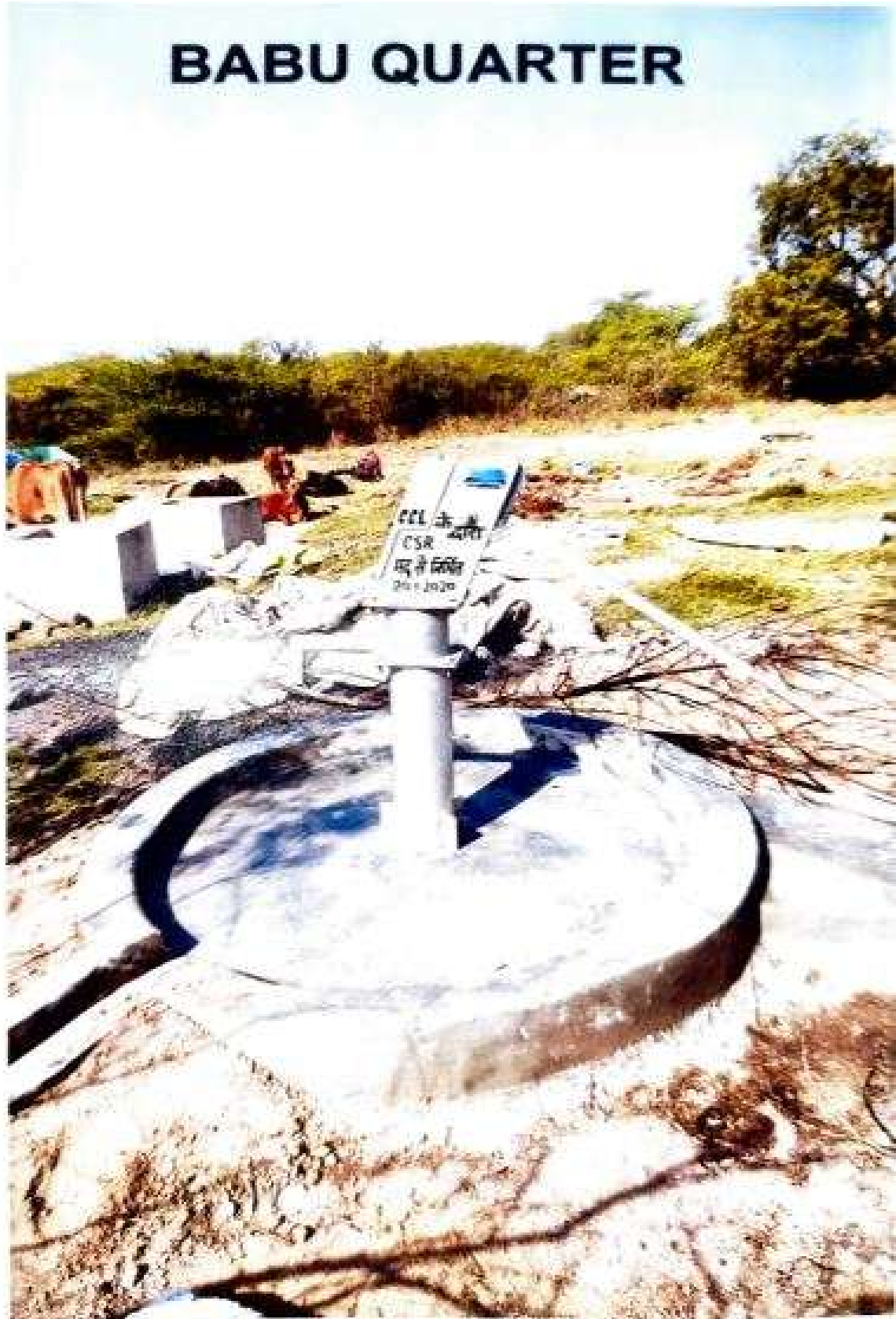
Figure 3: Handpump near Babu Quarters, Jarangdih
