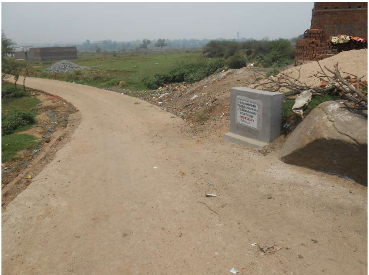
Figure 11: PCC Road at Patwa Basti, Hazari Panchayat
