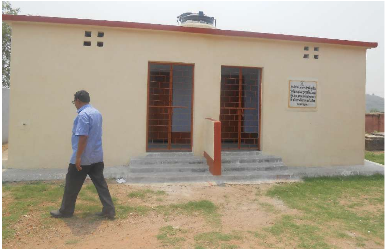
Figure 12: Construction of Toilets at Utkramit Vidyalaya, Turi Tola, Kathara
