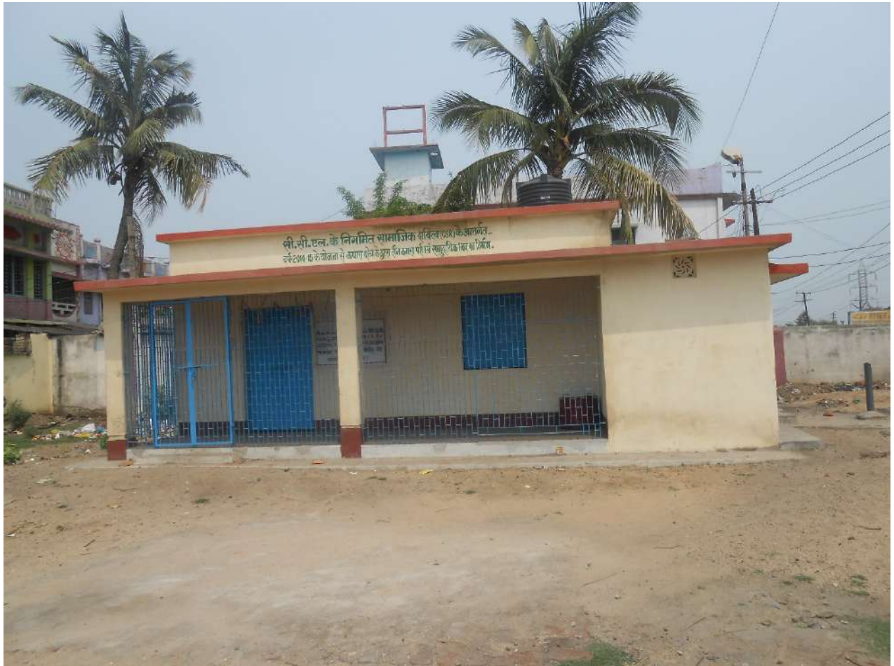
Figure 9: Construction of Three Rooms, Floor and Community Hall at Kathara
