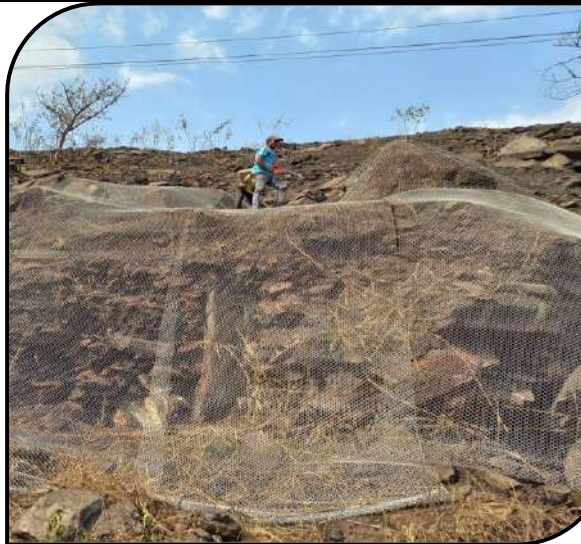
Photo-01 (Stone support of slope with wire-mesh)
