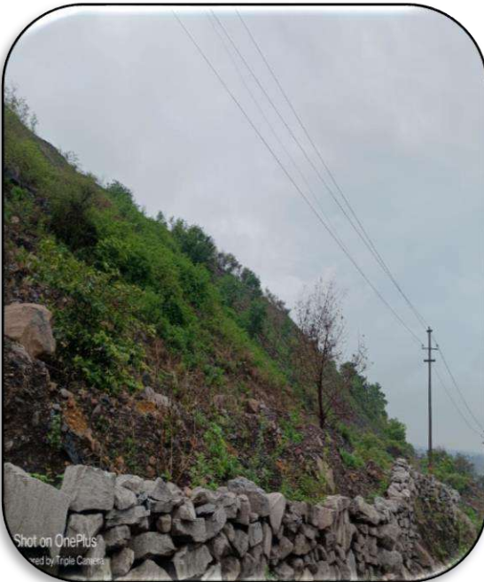
Photo-40 (Retaining/Toe wall along the OB Dump in east side)
