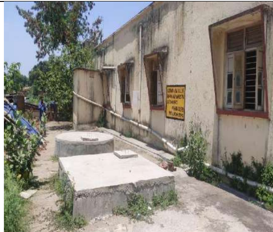
Photo-10 (Rainwater harvesting at PO Office)
