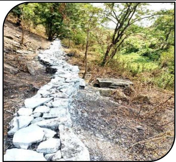
Photo-02 (Retaining/Toe wall along the OB Dump)
