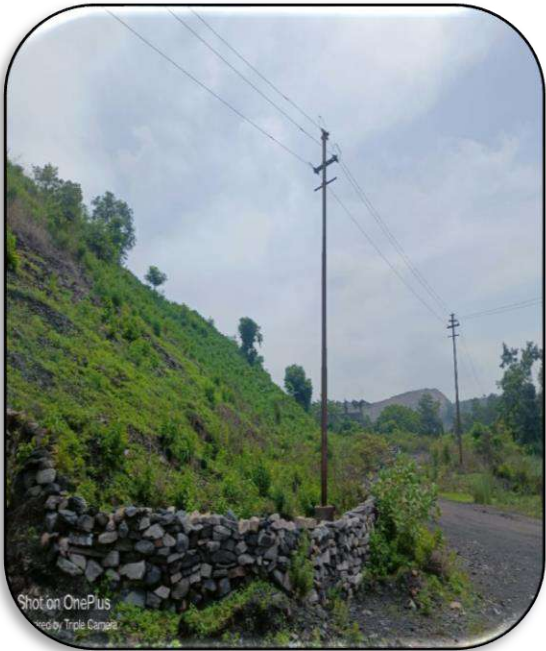
Photo-36 (Retaining/Toe wall along the OB Dump)
