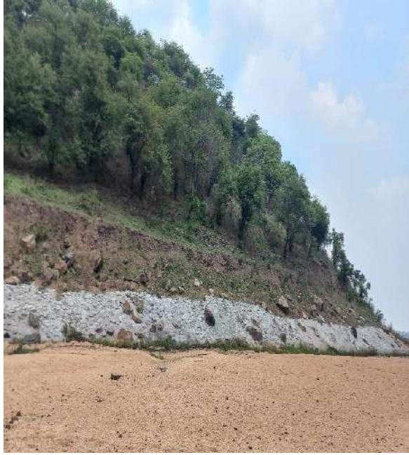
Photo -51 (Stone Revetment along Riverside)
