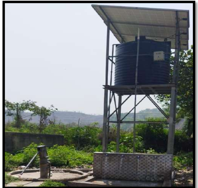
Deep Borewell at Kathara OCP
