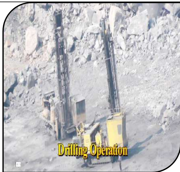
Photo-12 (Wet Drilling)
