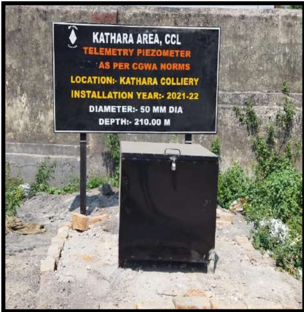
Piezometer at Kathara OCP
