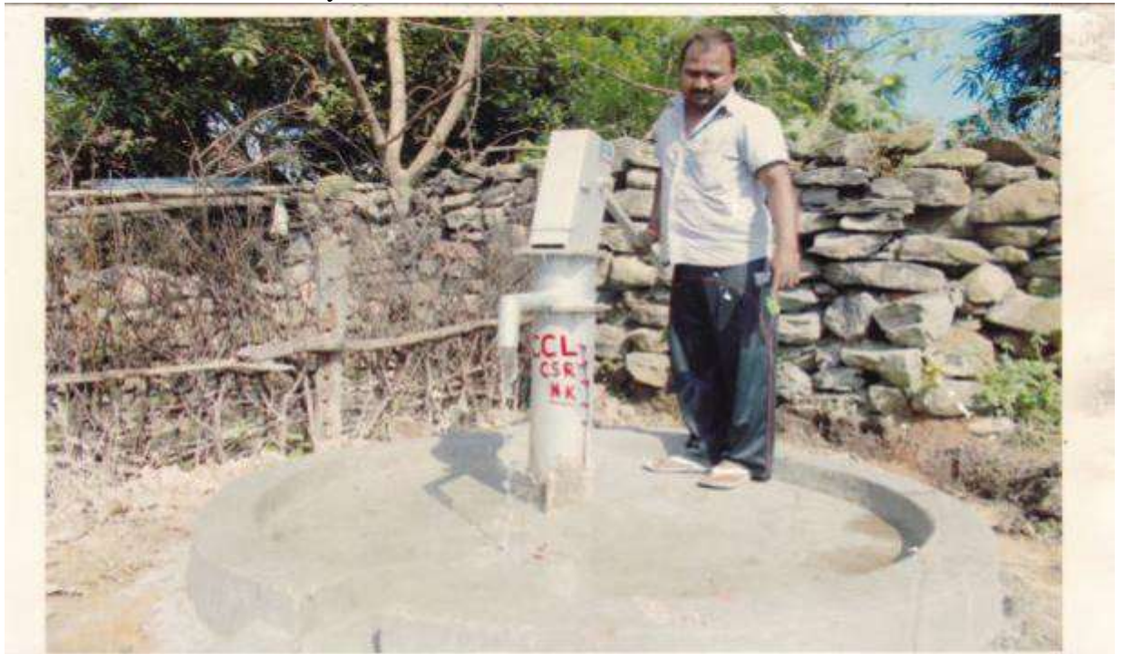
Installation of Hand pipes
