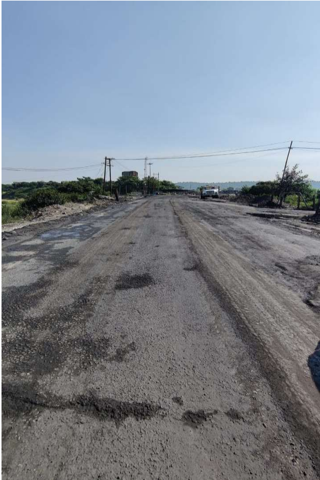
Figure 1.12 approach road to Dakra Siding
