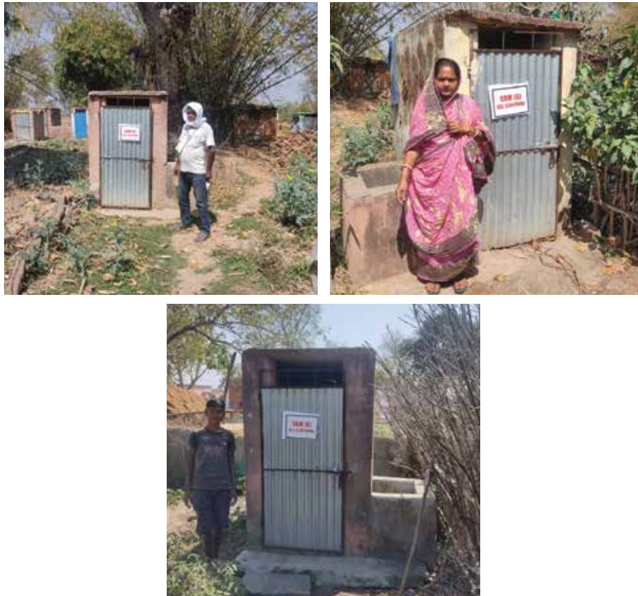
FIGURE 28: Constructed IHHL for Open Defecation Free Communities
