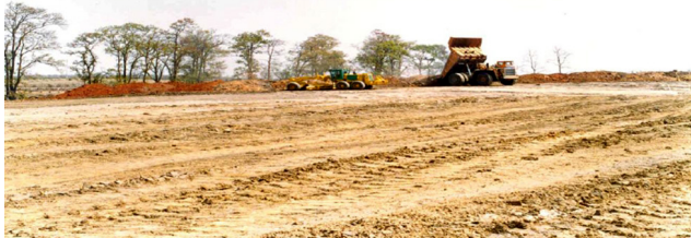
Spreading of Top Soil over back filled material
