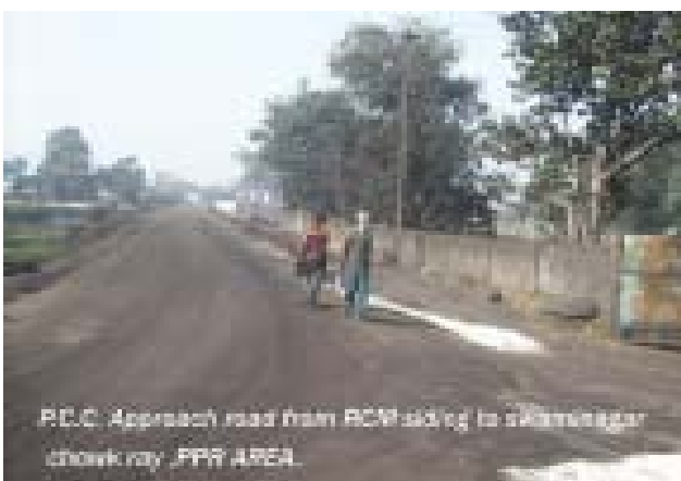
PCC approach road from RCM siding to Swaminagar Chowk, Piparwar Area
