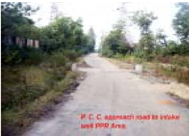
PCC approach road to intake well, Piparwar Area
