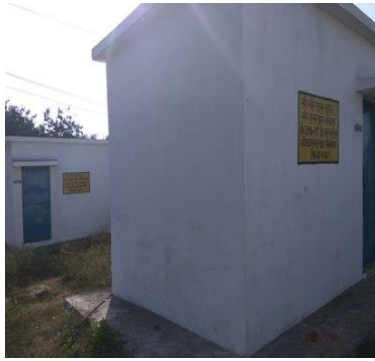
CONSTRUCTION OF TOILET IN PRIMARY SCHOOL NK
