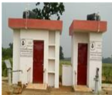
TOILET PIC HENGIR ODISHA PS BAUNSADHIA
