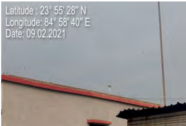
Continuous PM10 analyser installed at Railway Sidings of CCL
