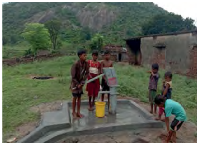
Handpump installed at Birhor Basti, CRS Barkakana
